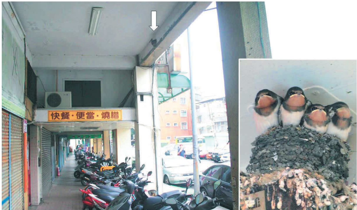
Fig. 1. A typical porch (or colonnade) of a Taiwanese city house in Xinyi District, Taipei. The vertical walls inside these colonnades are preferred nesting places for swallows (white arrow). Insert: Four barn swallow nestlings a few days before they fledge (16 May 2013). Photos taken by the first author.
